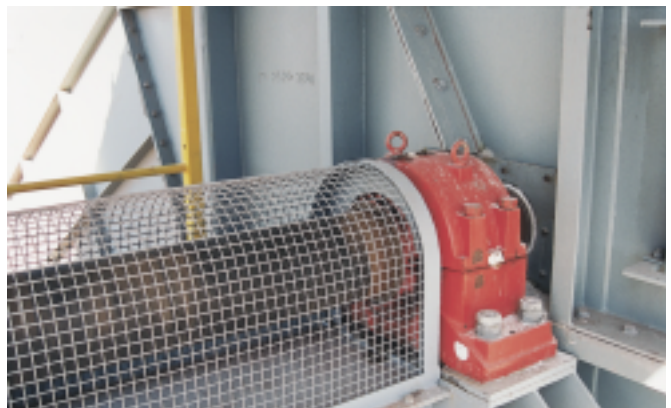
Ventilator drive unit
